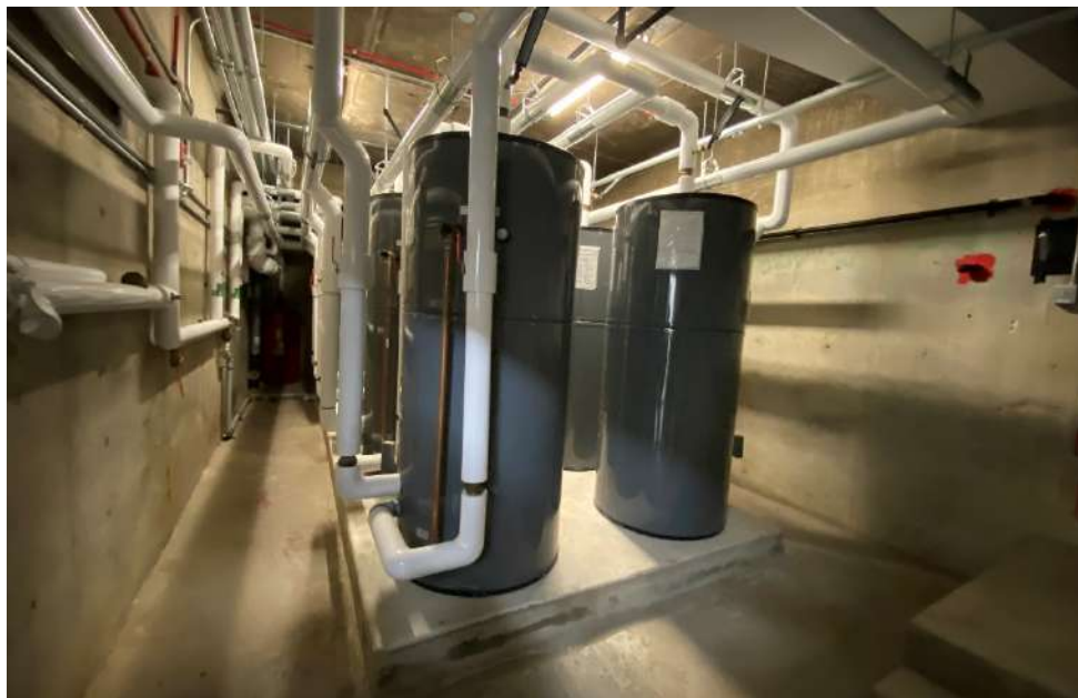
Photograph 24 – Interior, basement boiler room
