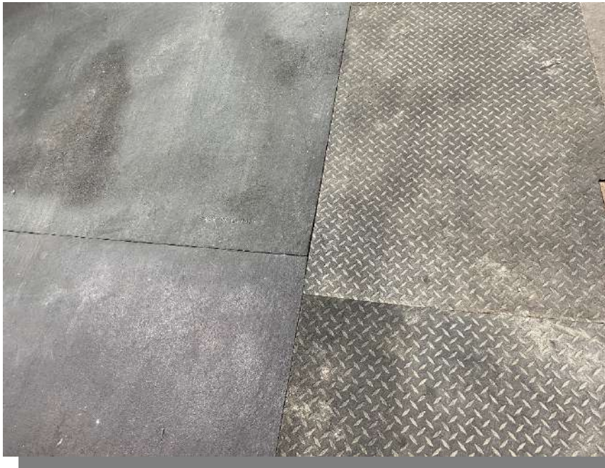
Photograph 34 – Interior, Arena flooring
