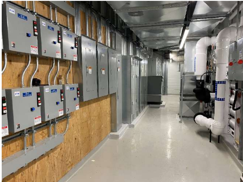
Photograph 28 – Interior, mechanical and electrical room Looking inward at the back area of the newly renovated mechanical and electrical room.
