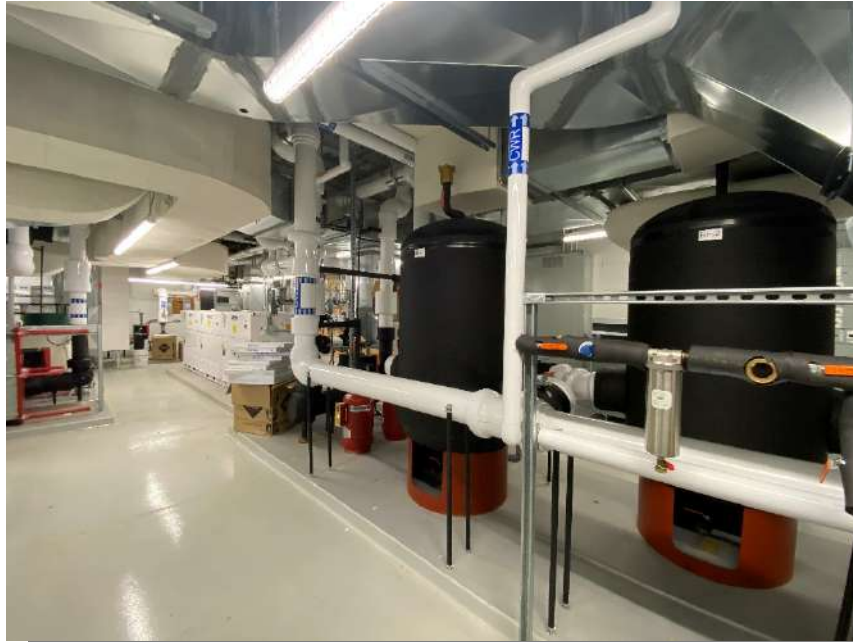
Photograph 27 – Interior, mechanical and electrical room Looking inward at the newly renovated mechanical and electrical room.
