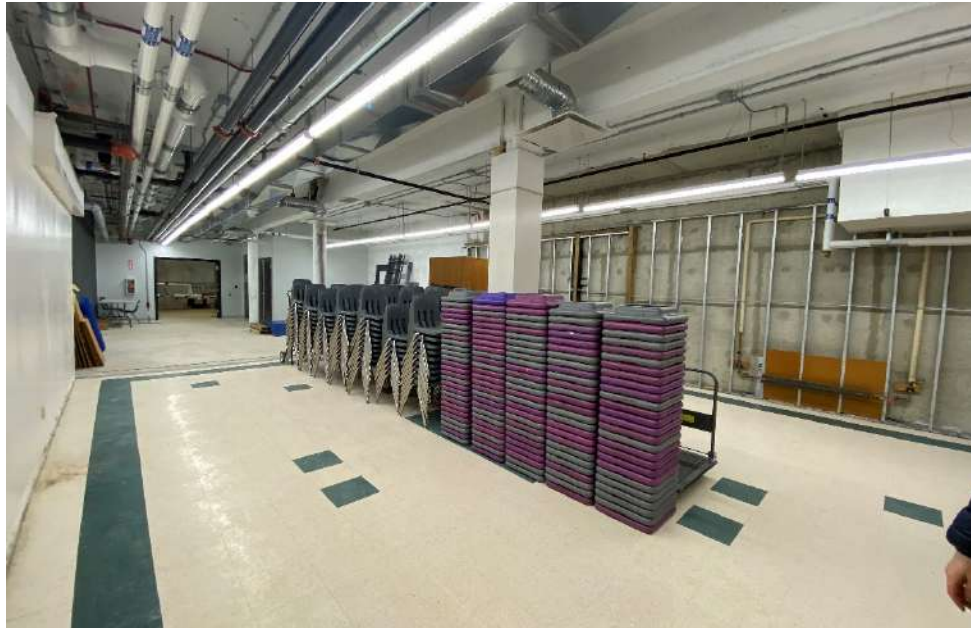
Photograph 23 – Interior, basement storage room
