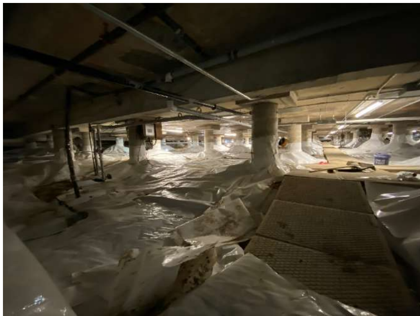
Photograph 32 – Interior, Arena crawlspace
