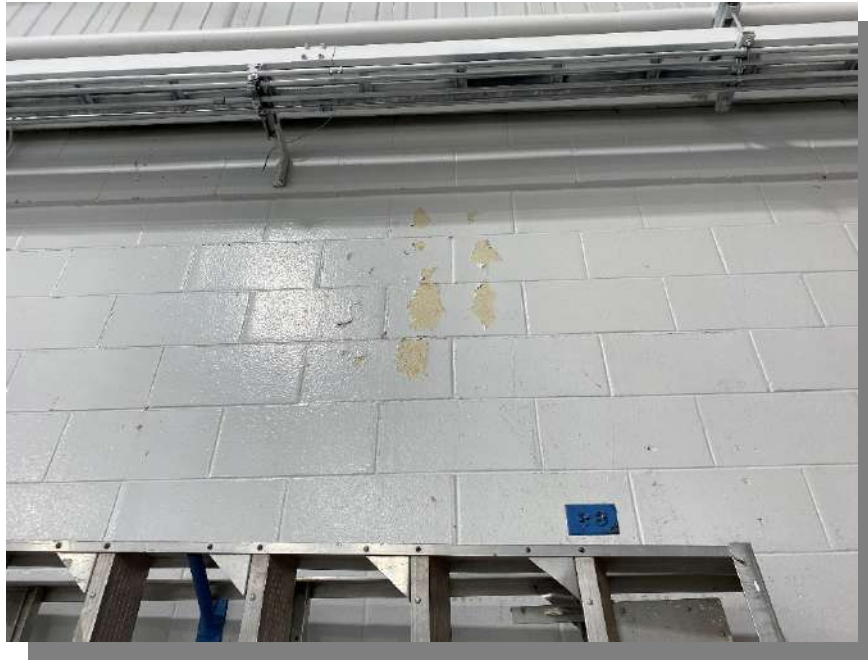
Photograph 35 – Interior, Arena north wall
