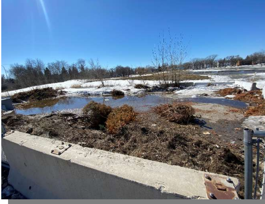
Photograph 47 – Exterior, stormwater catch basin
