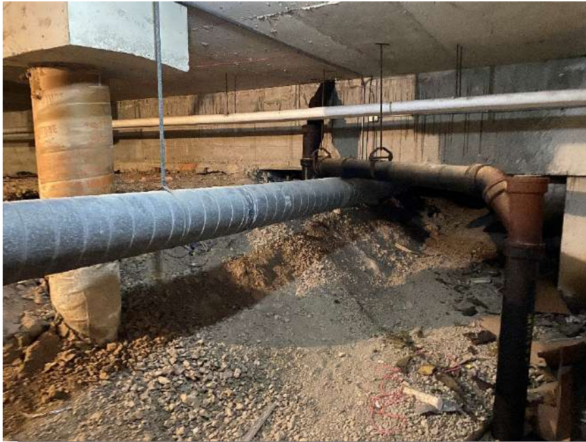
Photograph 33 – Interior, pool crawlspace
