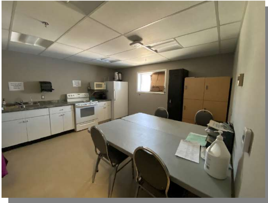
Photograph 21 – Interior, staff kitchen Looking inward at the staff kitchen (to be removed), north off the east corridor.
