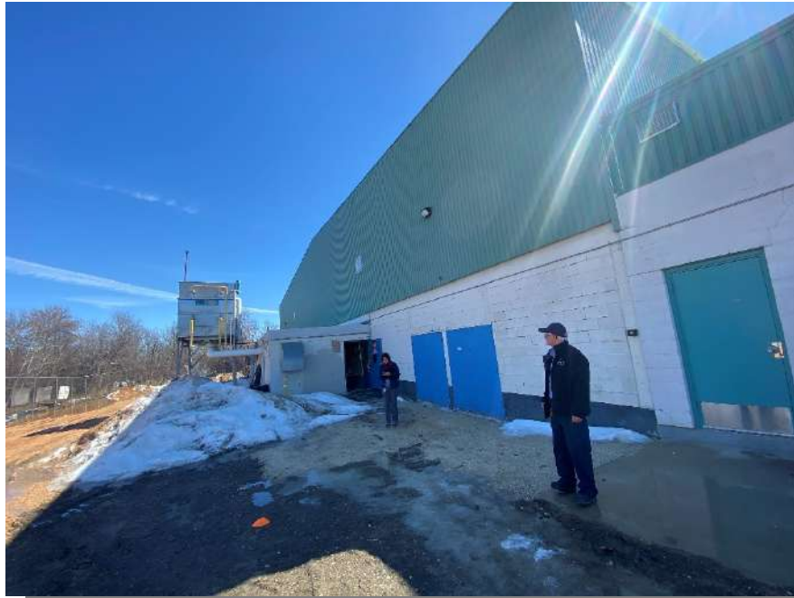
Photograph 7 – Exterior, north site boundary Looking southeast from the north elevation.
